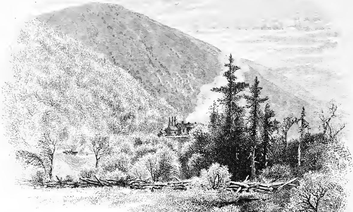
Hoosac Mountain and Tunnel Works.
